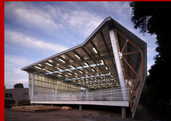
Box Hill Institute Trades Facility
